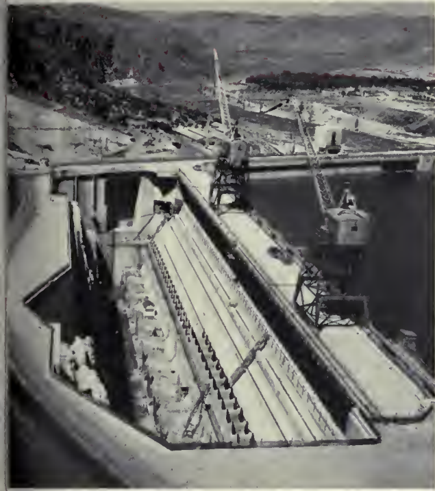
BEFORE AND AFTER —The world's largest pump is inside the 600-foot-long wing dam, adjacent to the left abutment of Grand Coulee Dam. The first view (above) was taken by F. B. Pomeroy on June 28, 1948, before the Morrison-Knudsen Co., Inc., and
